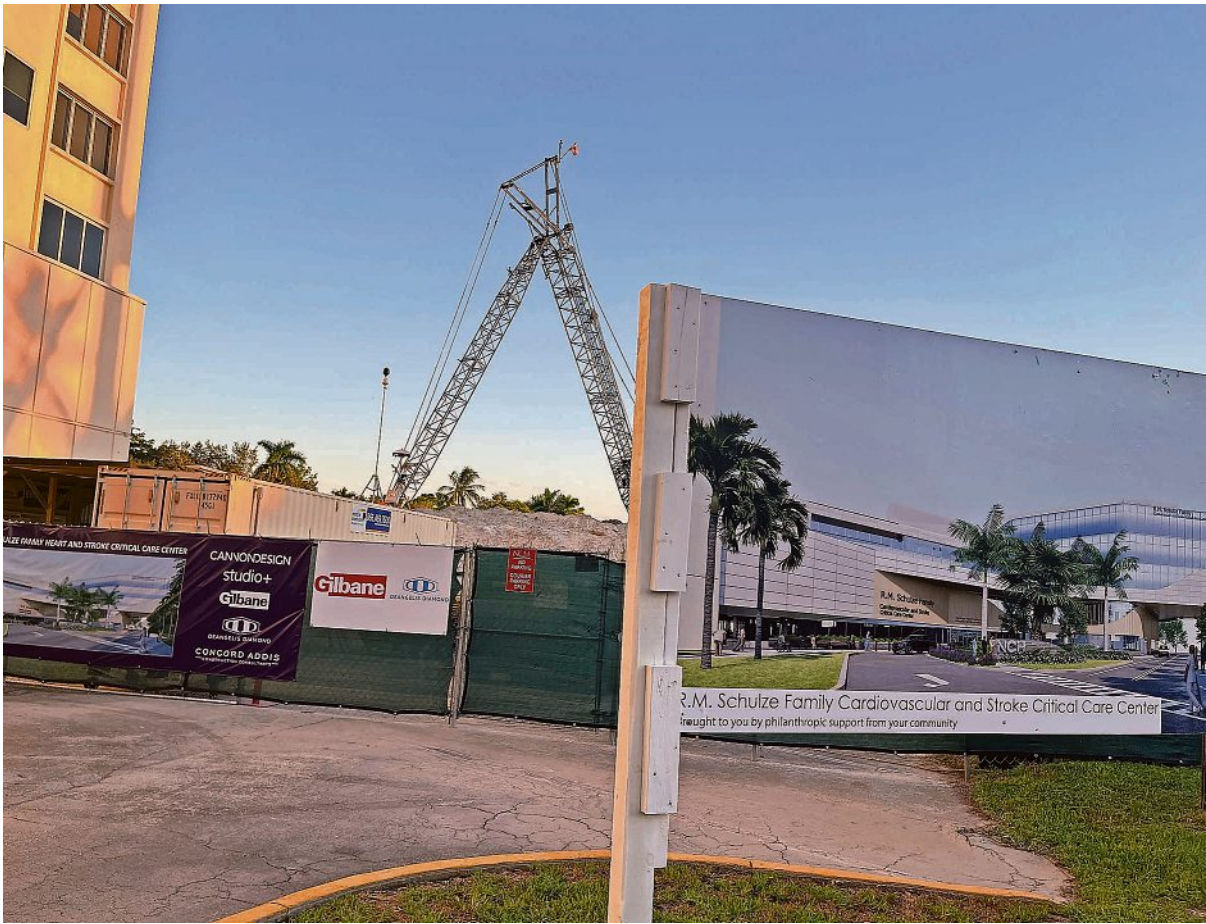
Construction site for NCH’s cardiac and stroke center on the campus of NCH Baker Hospital. Groundbreaking for the $295 million project was in June. The project is expected to take two years.
